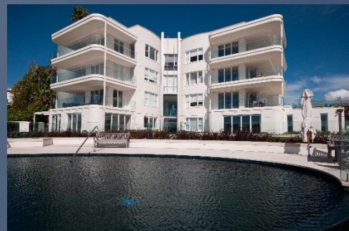
Remedial – Alterations & Additions
